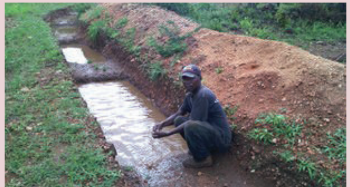
Water harvesting earth dam dug in the arable land Photo by: Nelson Mudzingwa
